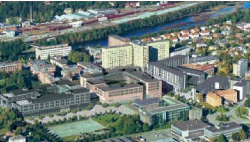
The hospital of the future relies on Swisslog logistics solutions: St. Olav's Hospital, Trondheim, Norway, as it will appear in the morning of August 7 th , 2006.
