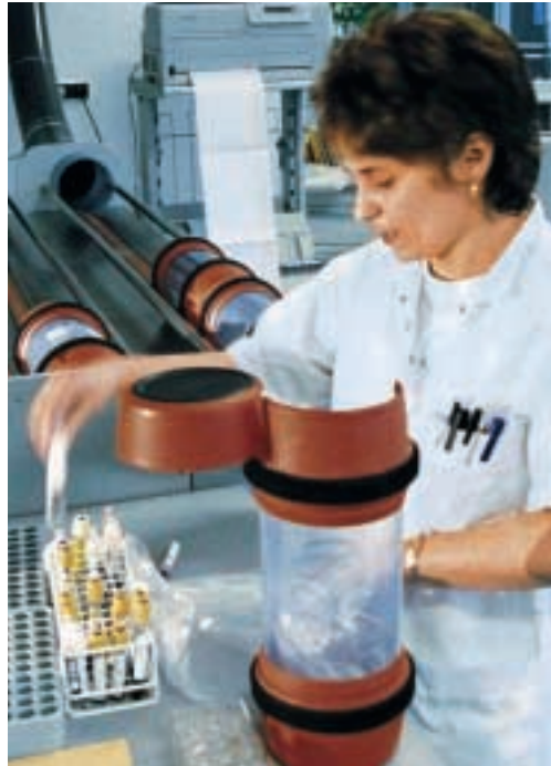
Swisslog's flexible pneumatic tube systems transport sensitive goods such as blood bottles or tissue samples in hospitals.
