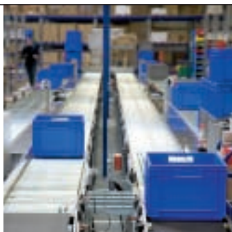
Modern conveyor technology provides for a fast and safe transport of containers
