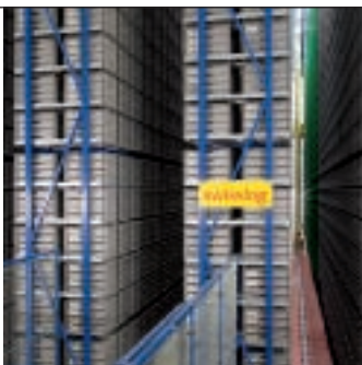
Front view of fully automated high-bay warehouse at SIS in Olten (Switzerland)
