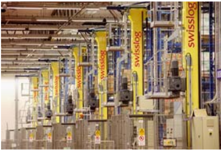
Swisslog-Accalon, Boxholm Pallet crane production
